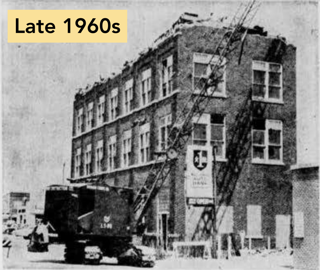
TALLEST BUILDING COMES DOWN
